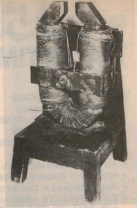
Shown at left is the "Electric Egg" used by Faraday for studying discharge phenomena in gases. At right is a close-up of Faraday's "great electromagnet". It was made from a section of ship's anchor chain, supported by a wooden stool.
