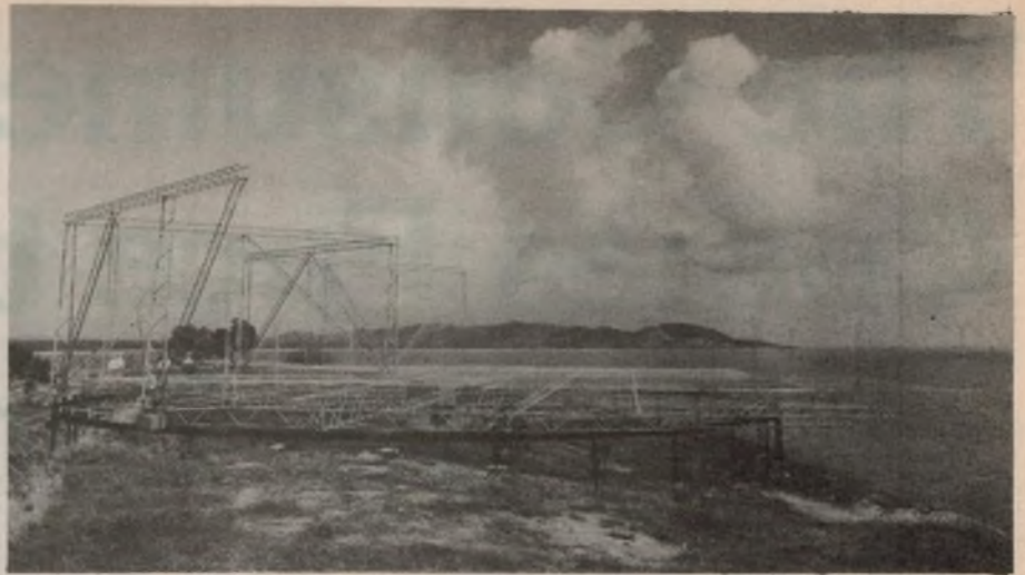
Fig. 1: General appearance of the Long Range HF Ocean Radar, Townsville, Qld.
