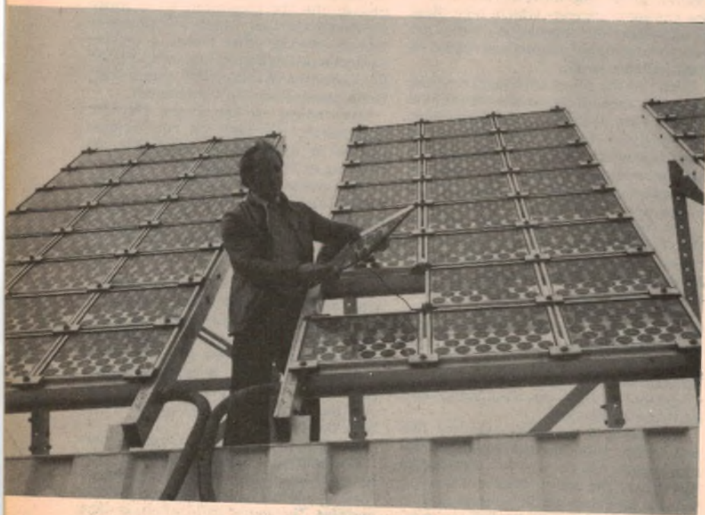
STO 3 Lyle Perkins displays a module of the 650 watt solar energy array mounted atop a standard shipping container. The container serves a dual role by also housing the recording instruments and storage batteries.
