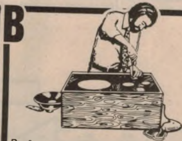
B: Screw in the speakers and wire them as shown in the detailed instructions. A pre-assembled 'loom' is supplied -- no soldering required.
