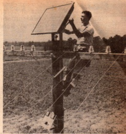
Above: Solar power installation for remote area communications. Left: Typical 12V 7.2W solar cell array.
