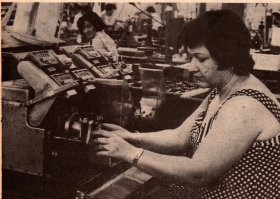
Pictured above is the older method for winding transformers. Miss Barbara Dickson hits the button on the "stick" winder to wind 10 coils simultaneously. Meanwhile, below, Mrs Vicky Tsiganos works on the newer method with the large bobbin winder. Transformers now account for about 20% of A&R sales.
