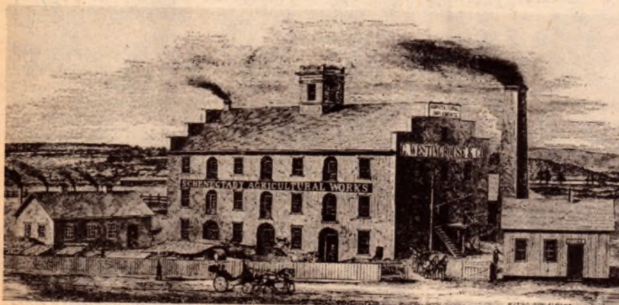
Where George Westinghouse learned his trade — the factory of the elder Westinghouse in Schenectady, New York. The factory started in 1856.
