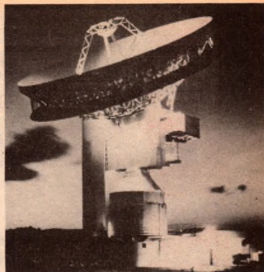
Sending to the sky, the giant (30-metre diameter) antenna at Cayey, Puerto Rico, relays messages overseas via Intelsat. Most earth stations are this size.
