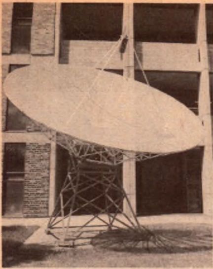
ABOVE & RIGHT: Two views of the 5-metre parabolic dish antenna.
