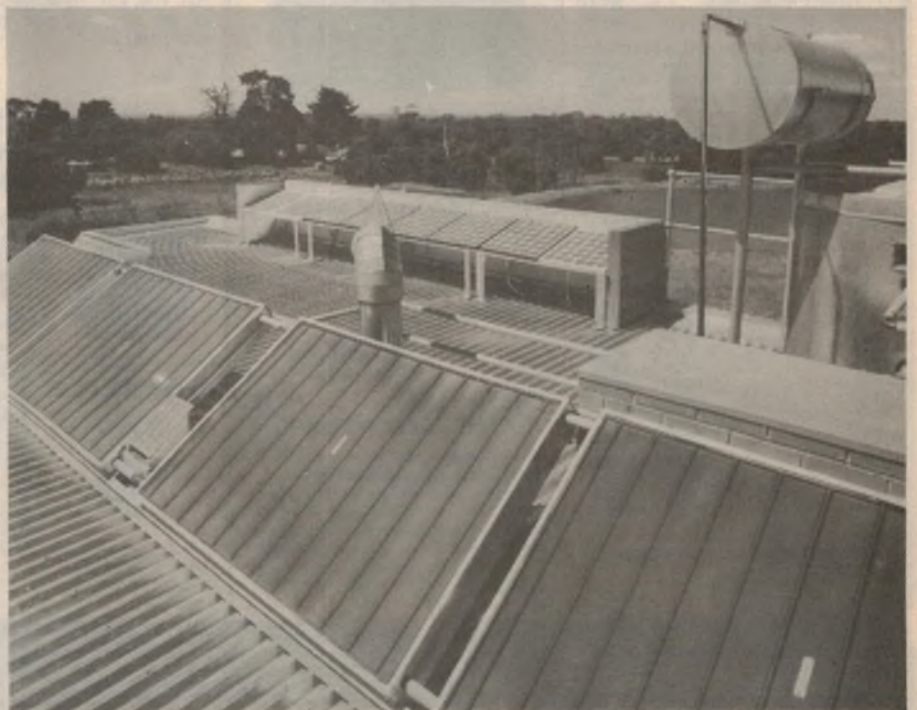
Rainwater is collected from the roof for domestic use and heated by conventional flat plate solar collectors. Hot water is stored in a roof-mounted 730 litre tank.
