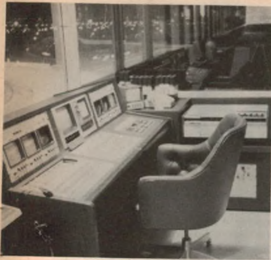
The control centre for the display board at the New Jersey Meadowlands Racecourse. Pre-recorded messages and animated entertainment features can be shown, as well as scenes from other sporting events and vital photo-finish shots.
