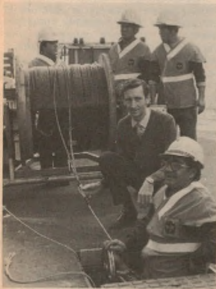
Cable laying required special equipment
