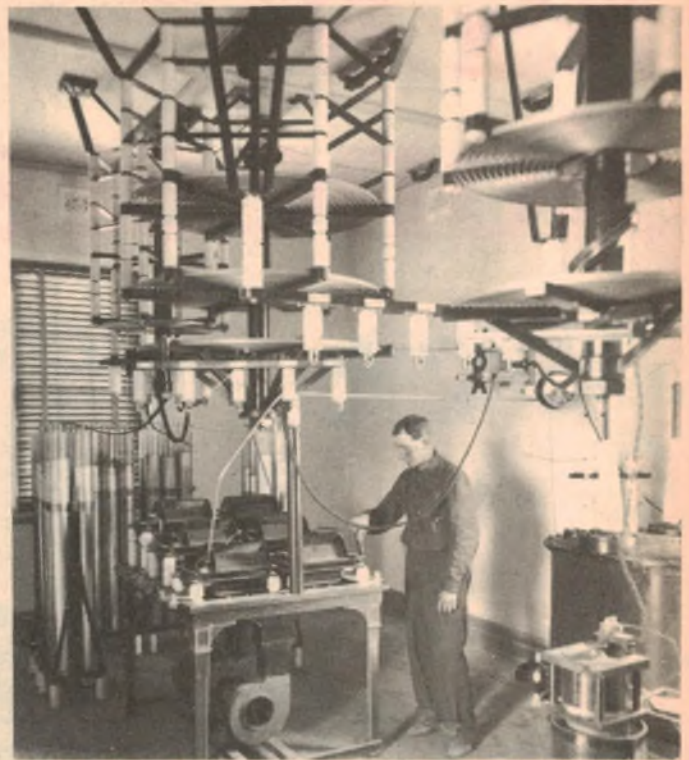
The high tension room at the Pennant Hills station, showing the original Telefunken equipment installed by Australasian Wireless Ltd.
