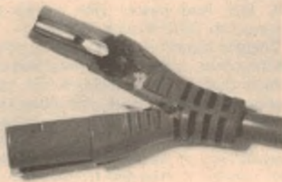
The faulty power plug. The pocket of carbon adjacent to the inner end of one of the pins is clearly visible.
