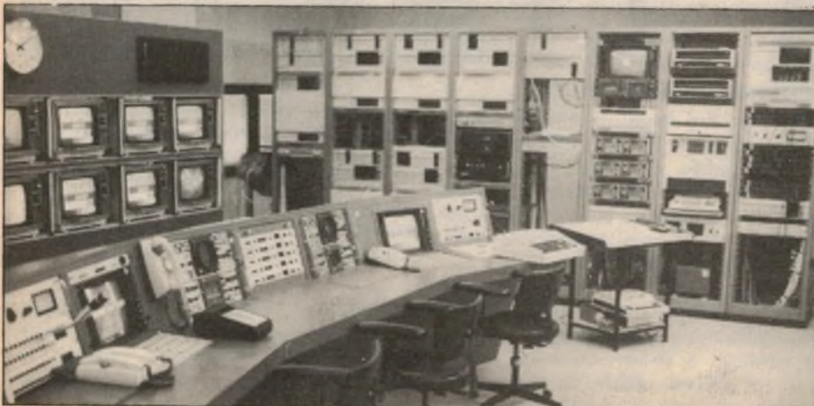
Above: The ABC Games Unit television packaging suite. In the immediate foreground is the audio mixer and at the far end of the bench is the vision mixing console. Also visible are eight one-inch video tape machines made by Ampex. Below: The central apparatus room where incoming and outgoing signals were switched and synchronised.
