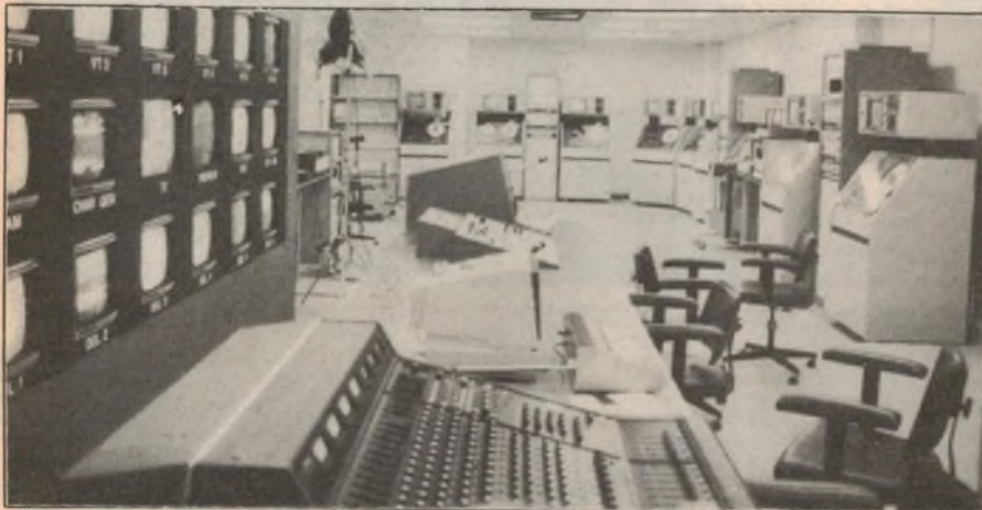
Above: The ABC Games Unit television packaging suite. In the immediate foreground is the audio mixer and at the far end of the bench is the vision mixing console. Also visible are eight one-inch video tape machines made by Ampex. Below: The central apparatus room where incoming and outgoing signals were switched and synchronised.
