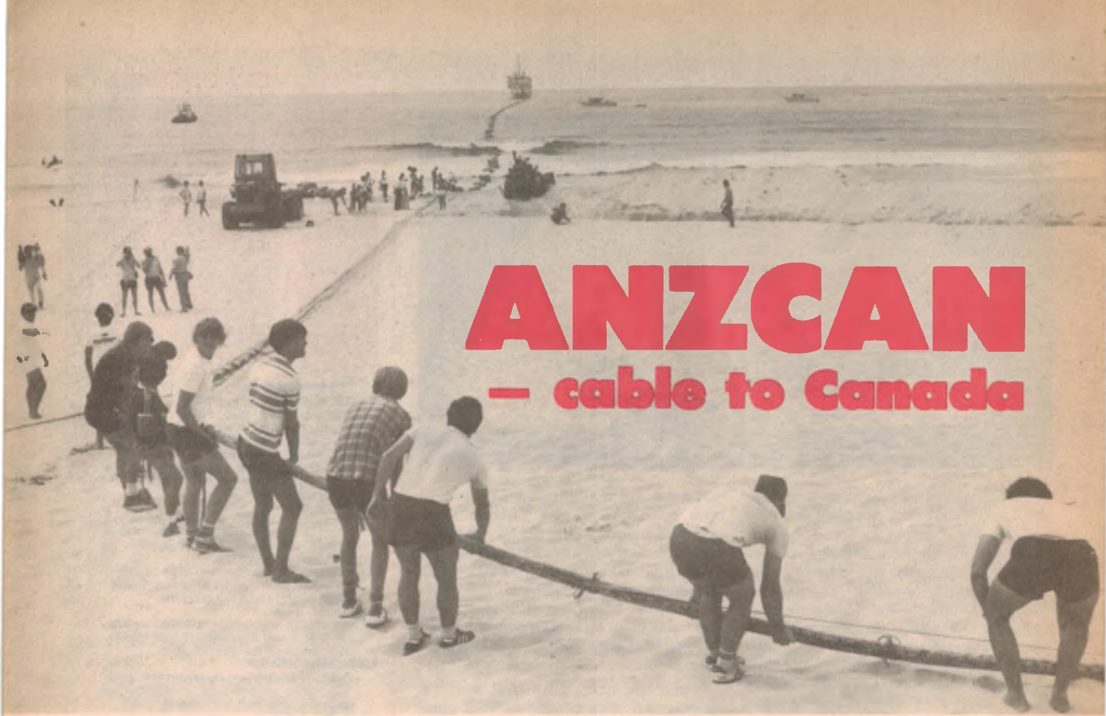
Bondi Beach. Volunteers prepare to lay the ANZCAN cable in the trench prepared for it, seen in the background.
