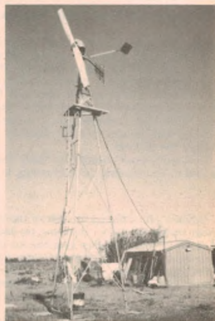
Wind powered generator system built by the author produces 250W in a 40km/h wind.
