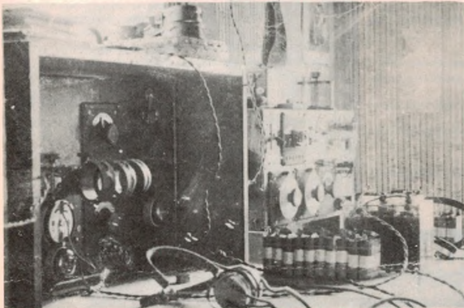
Honeycomb coil receiver at 2YK, New Zealand's first radio station.
