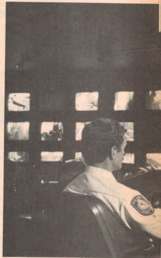
A portion of the SCATS Control Centre showing some of the 32 TV monitors, two of the control consoles, and a graphics display set suspended from the ceiling.
