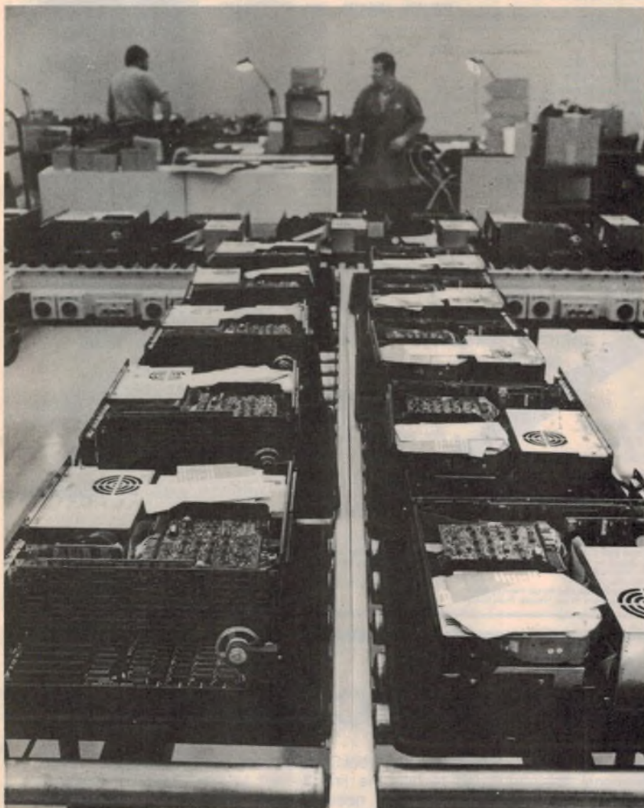
PCs plough down the line for run-in tests. At right, disk drives undergo testing with PC software routines.
