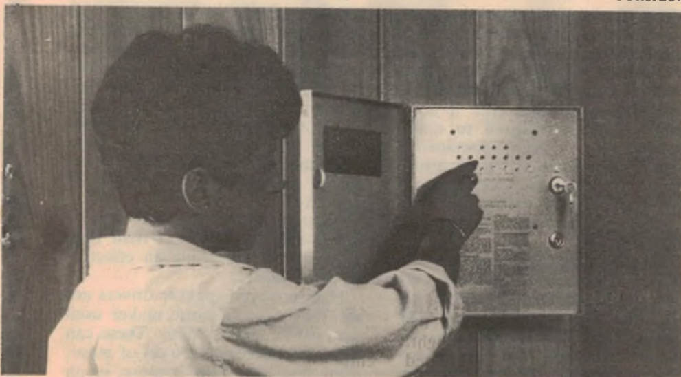
Figure 23. This control unit has an Automatic Digital Dialler built in.
