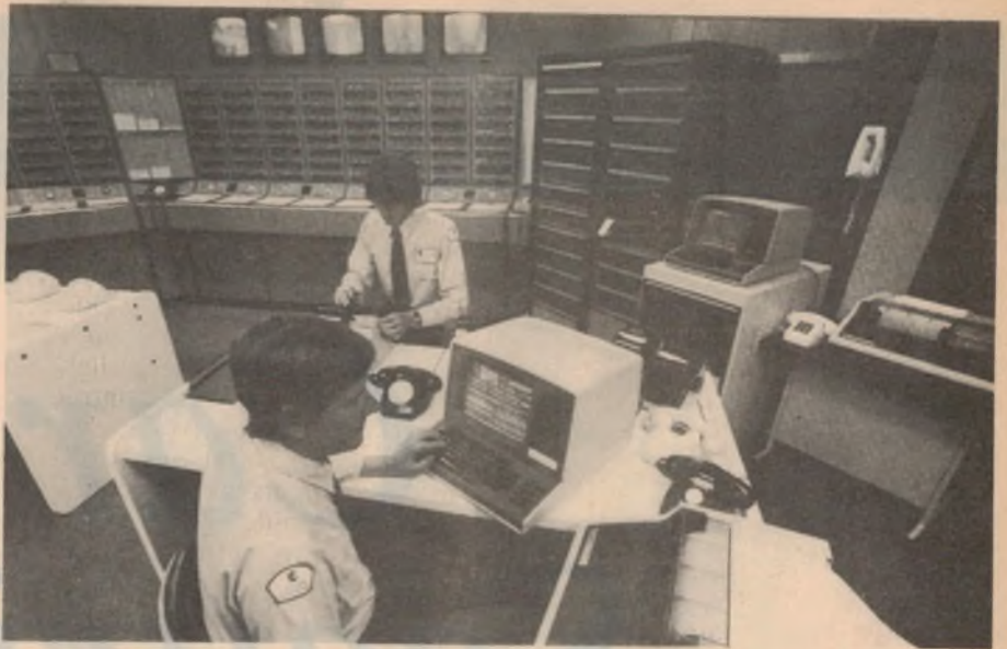
Figure 24. This central monitoring station can provide services from 24hr video surveillance of your home to notifying the police when an intrusion is detected.
