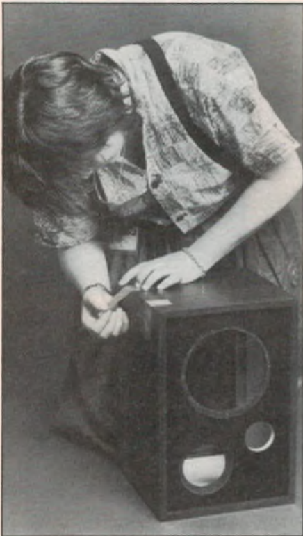
The assembled cabinet is held together by strips of masking tape until the glue dries. The woofer cutout is adjacent to the base board.
