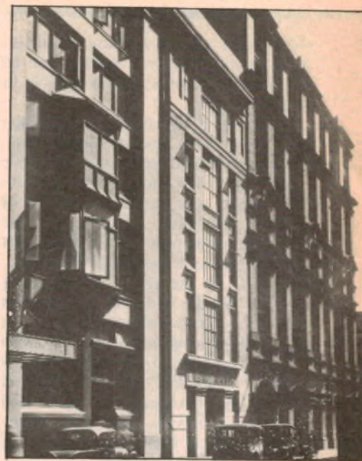
This view shows the main DC sub-station in Clarence Street as it existed during the 1930s.
