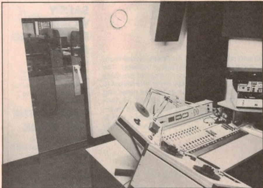
The heavy laminated glass door is the secret of success of the new studio construction technique. It provides a very high degree of acoustic isolation.
