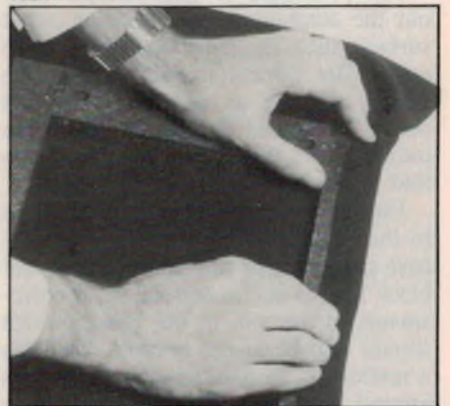
The grille cloth is stretched over the framework supplied and retained with tacks.
