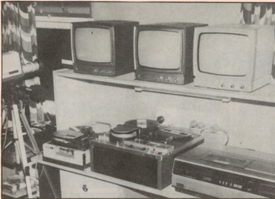
Showing the equipment set up in the "Editing" mode. The Portapak is on the left of the bench, then the 3670 editing machine and the VHS unit on the right. The three modified Kriesler monitors are on the shelf, and the AVC3420 camera on a tripod on the extreme left of the picture.
