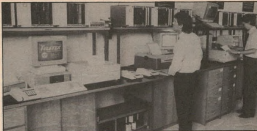
A complete terminal setup for ISDN, integrating telephones, fax, videotex and telex. (Courtesy STC)
