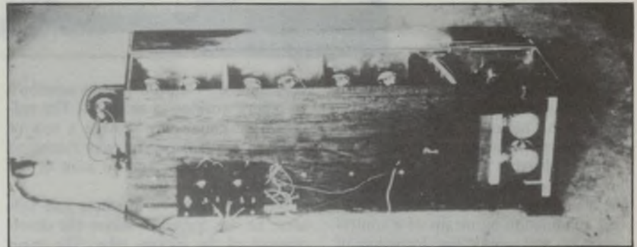
The multi-stage video amplifier, using valves, which Mr Takayanagi used in his early experiments around 1926-27.
