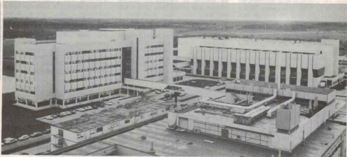
Taken at the Philips Research Laboratories complex in Eindhoven, this shot shows the new VLSI Design Centre on the left, and the Submicron IC Centre on the right.
