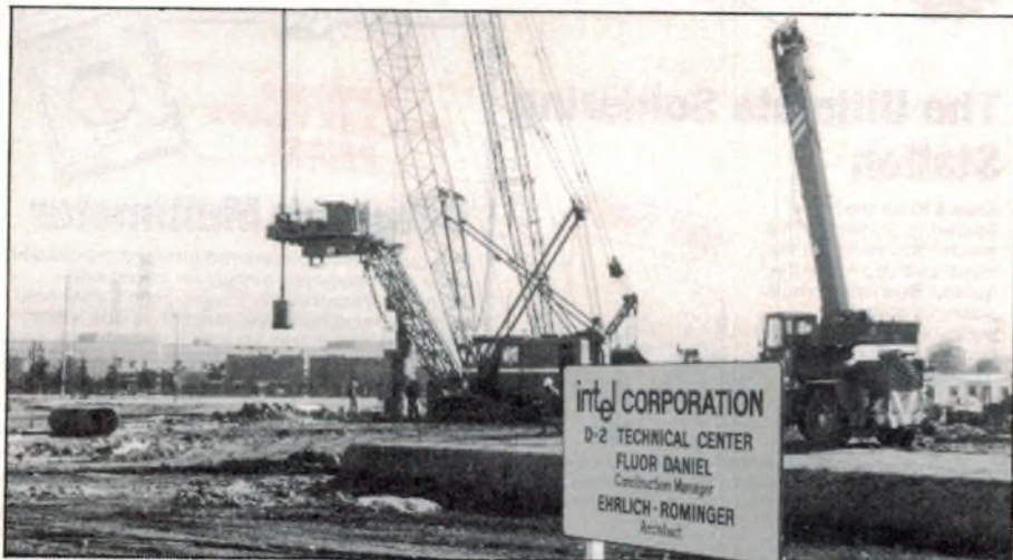
Construction begins on Intel's new facility
