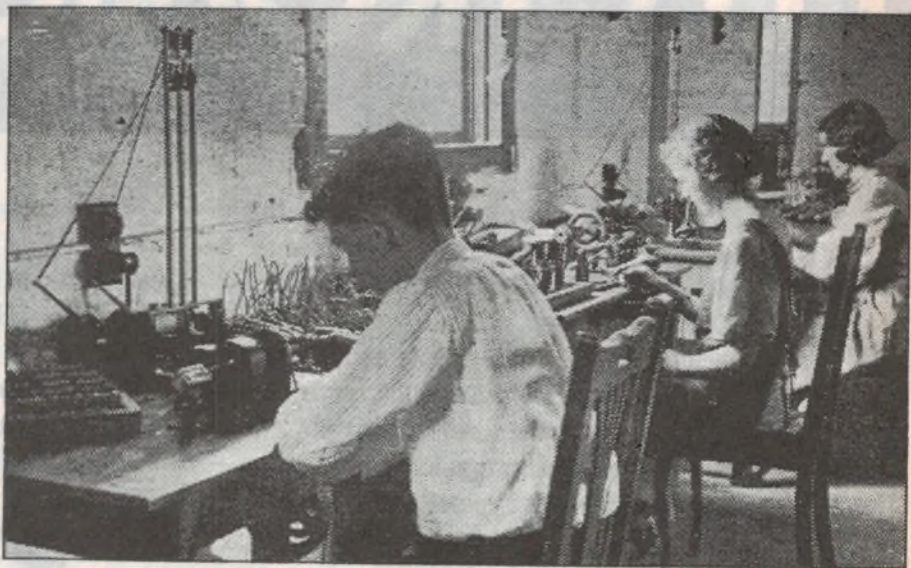
Winding coils at the Ivy Street, Darlington factory in 1934. A contemporary story noted that the factory could turn out 'several thousand coil units per day', with 40 different types of coil.
