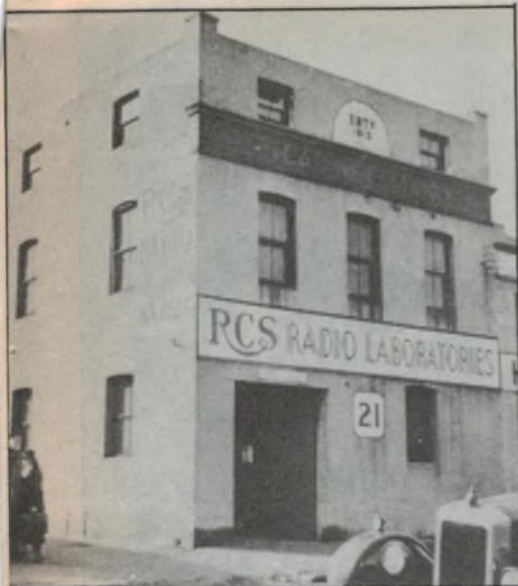
Front view of the Darlington factory, which was gutted by fire in July 1938.
