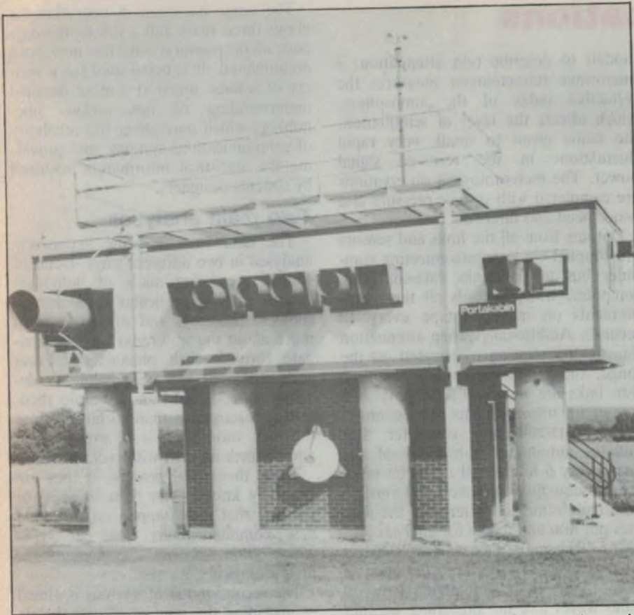
The transmitter cabin at Chilbolton. Hoods keep rain off the windows through which the signals are transmitted. The transmitters are mounted on benches supported independently from ground, inside the four concrete pillars. This prevents vibrations in the cabin affecting the equipment. The anemometer and vane mounted on top of the cabin measure wind velocity.
