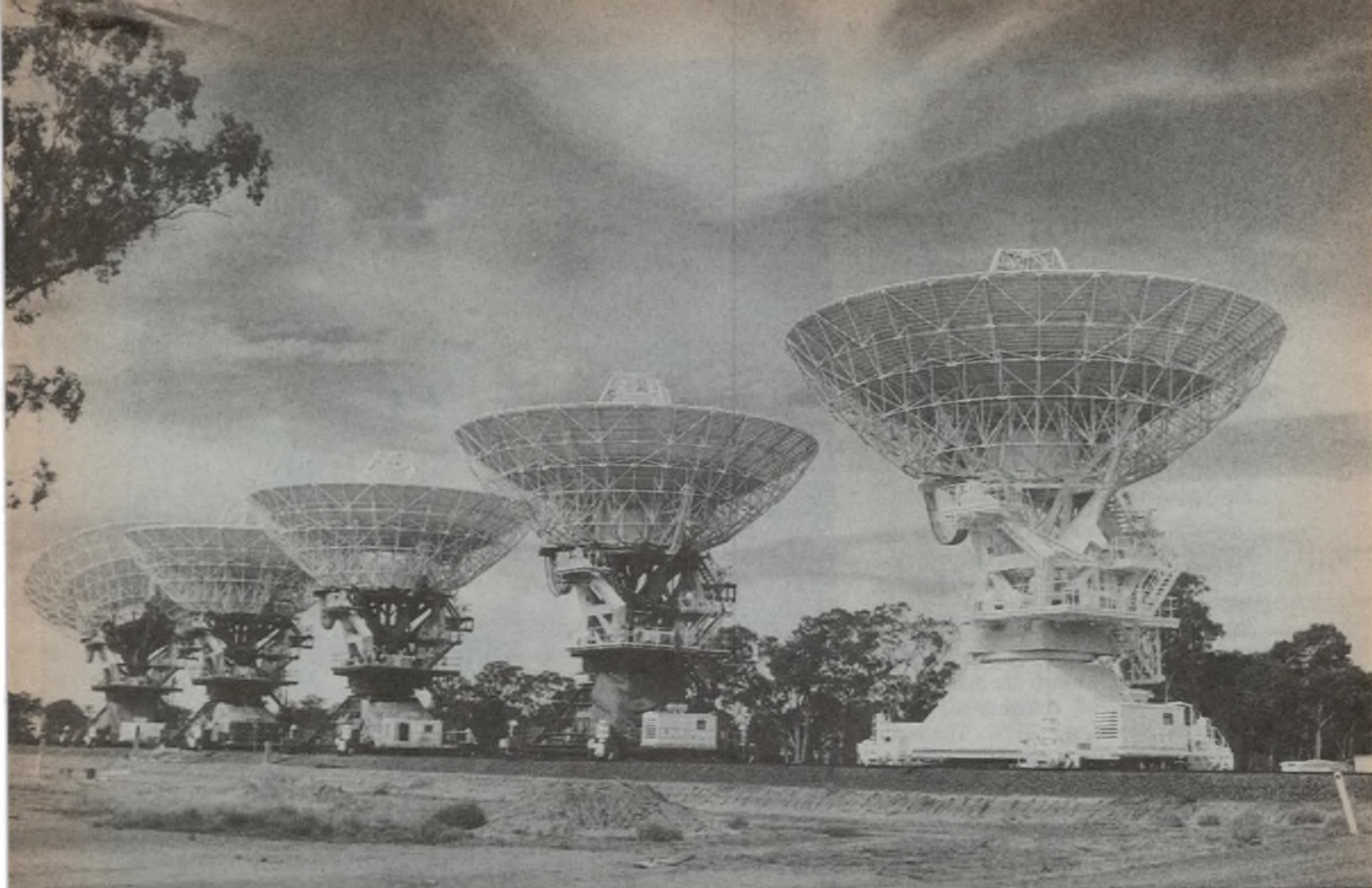
The five closely-spaced dish antennas at Culgoora, nearing completion. When finished and operational they will be deployed along 3km of tracks, with a sixth dish 3km further west.
