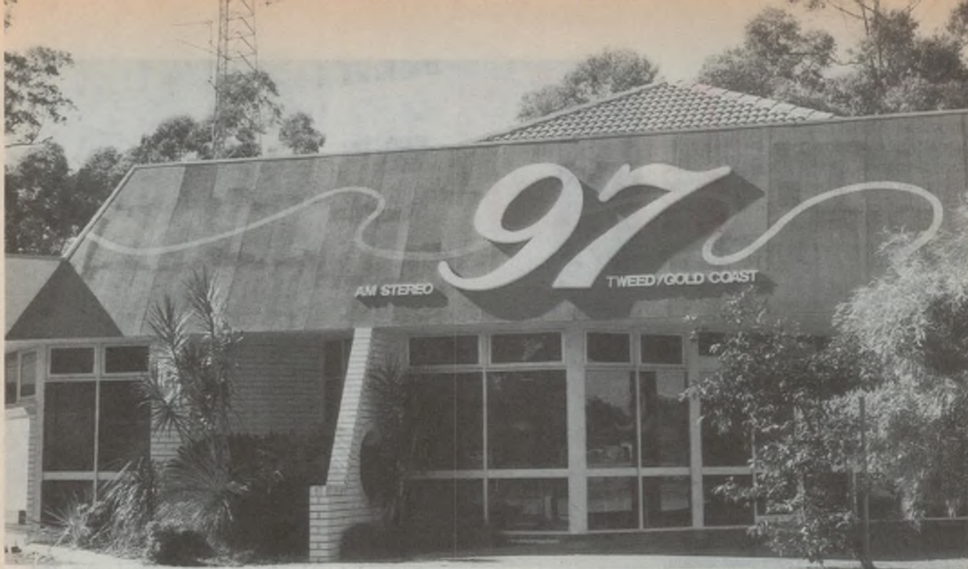
Outside the modern 2MW studios in Tweed Heads, with microwave uplink just visible at top left.
