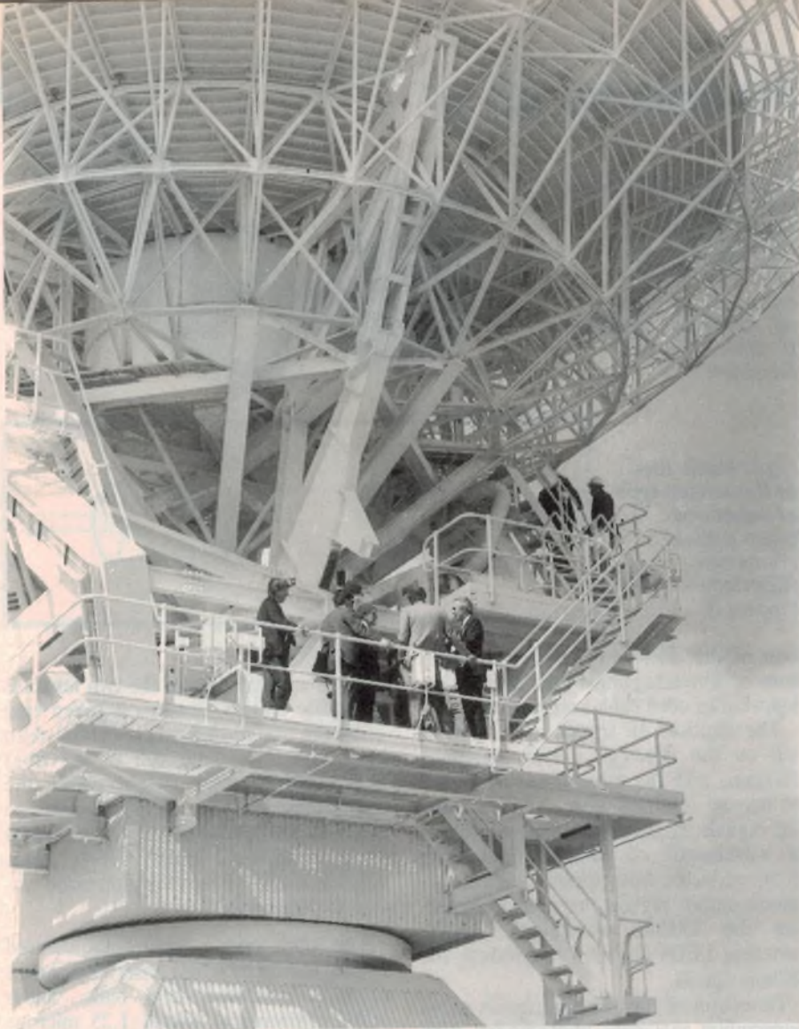
You can get an idea of the size of the dishes from this shot, looking up from trackside on the day the AT was officially opened.
