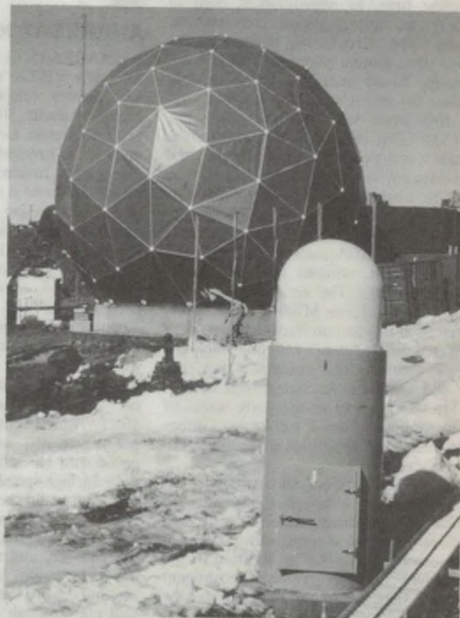
The completed ANARESAT radome at Mawson base. In the foreground is the Inmarsat terminal, which will act as a standby for ANARESAT.
