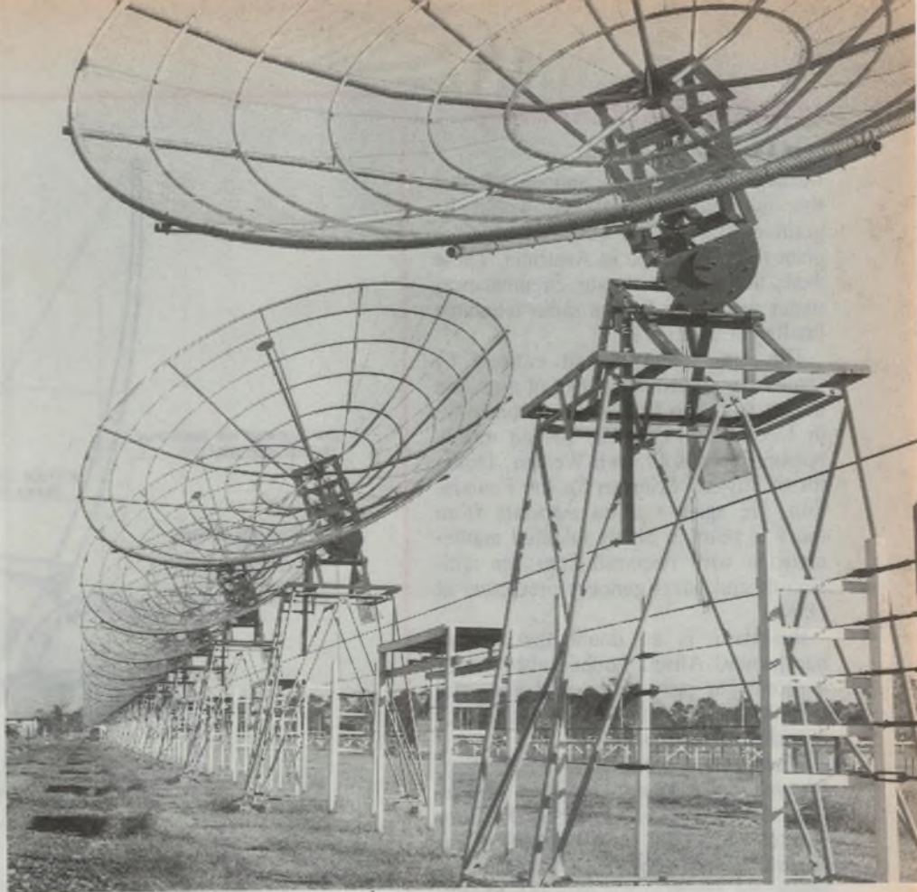
Fig.10: Closer view of the dishes forming the 1410MHz Chris-Cross array at Fleurs Field Station, built in 1957.
