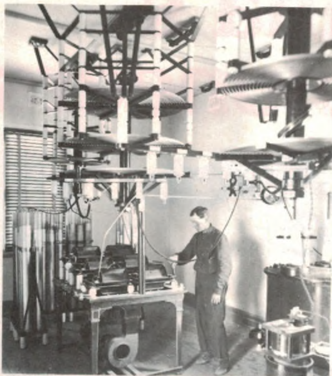
The high tension room at the Pennant Hills station, showing the original Telefunken equipment installed by Australasian Wireless Ltd.
