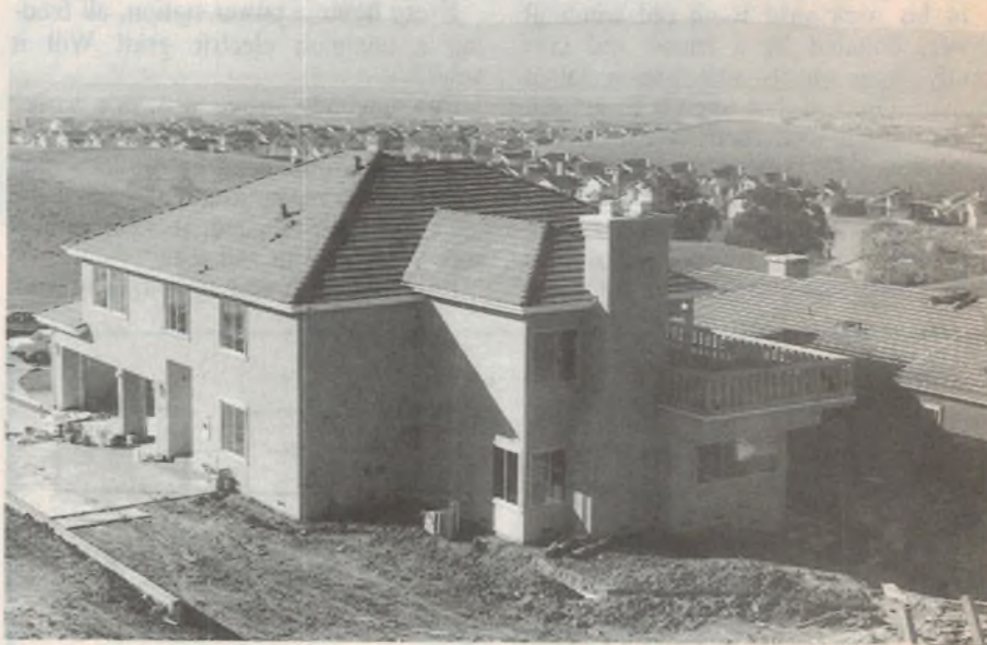
This new US$1.3 million home overlooking California's 'Silicon Valley' has been fitted with the new 'Home Manager System' developed by Advanced Security Engineering.
