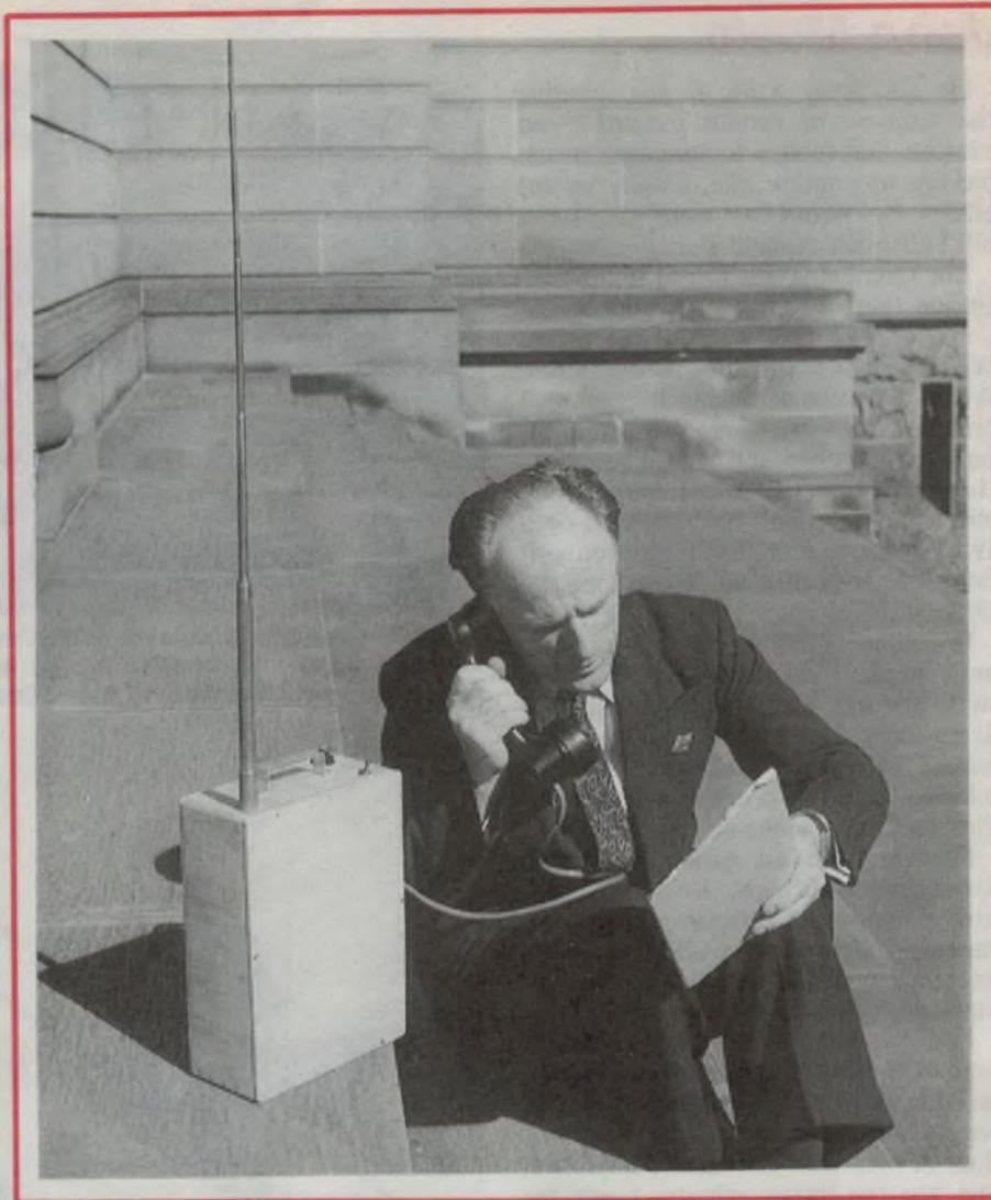
**A little further down the track, John tests a portable transceiver, one of several which he designed and produced in collaboration with the R & H staff. They could be used by reporters on foot, or in collaboration with news cars in remote areas. (Courtesy Dr Alice Moyle)**
