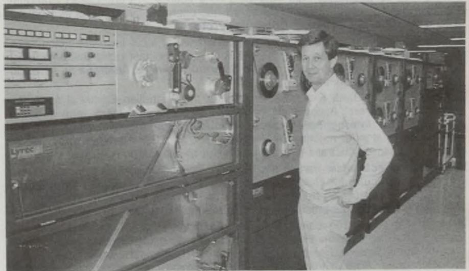
Festival Records has added a new Lyrec P-4400 'master loop bin' to its tape duplicating facility, a move which is capable of increasing production capacity by as much as twofold, according to Festival's Barry Nagel.
