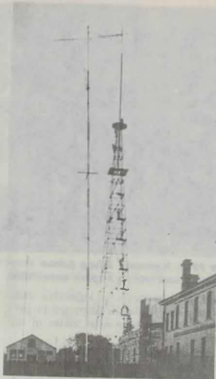
The 76m antenna tower and mast erected at the rear of 4 Dutruc Street, Randwick around 1911.
