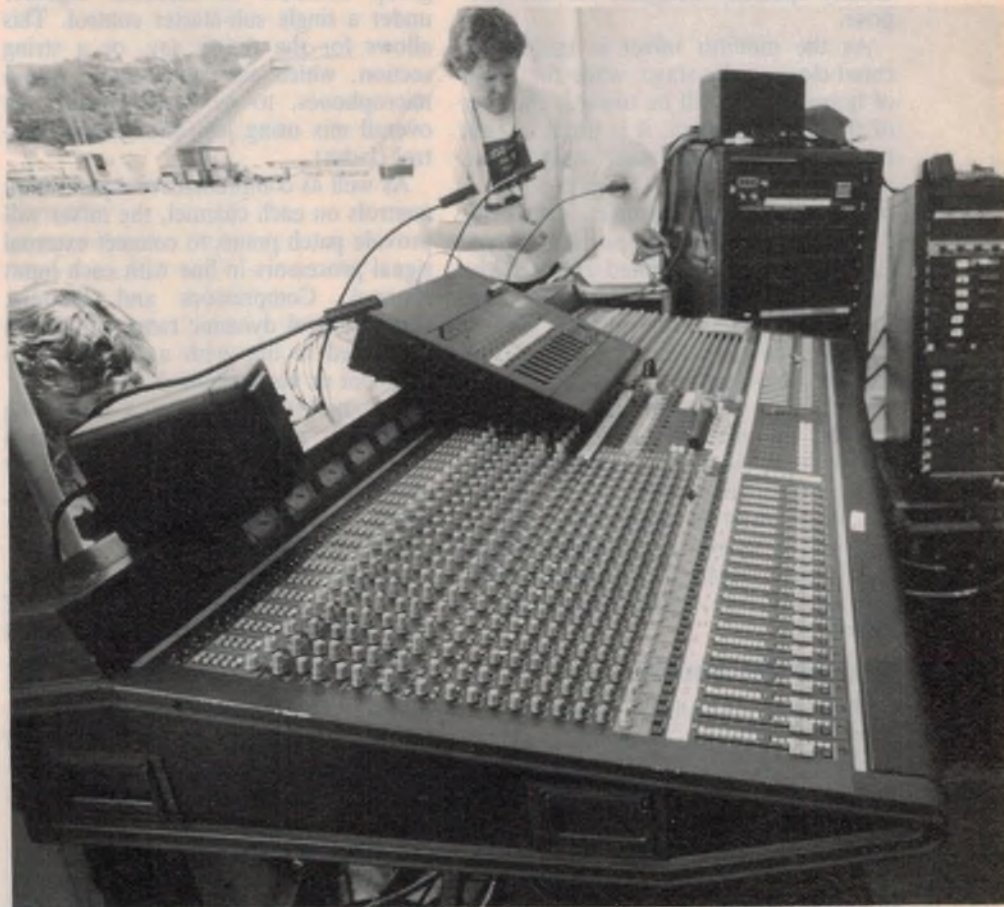
The front of the house mixer, with three racks of outboard signal processing equipment.
