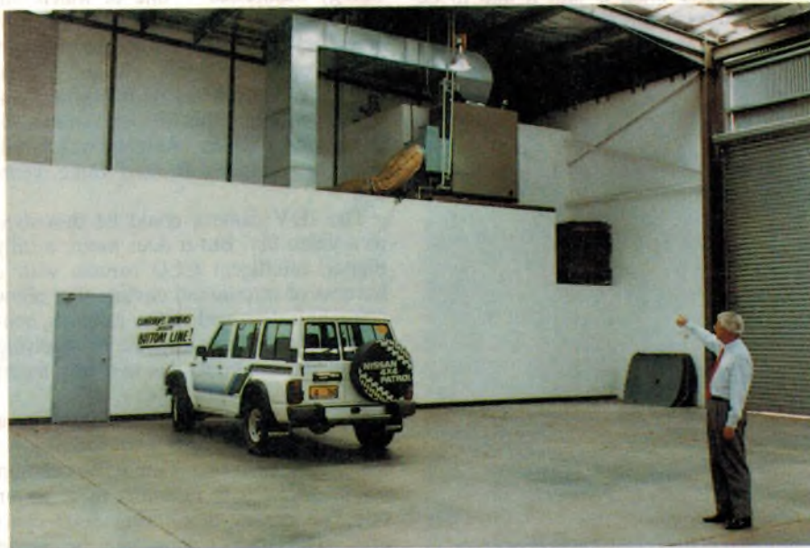
A typical warehouse installation showing how well the security camera can be concealed: the camera is at centre of picture directly above the car's spare wheel.
