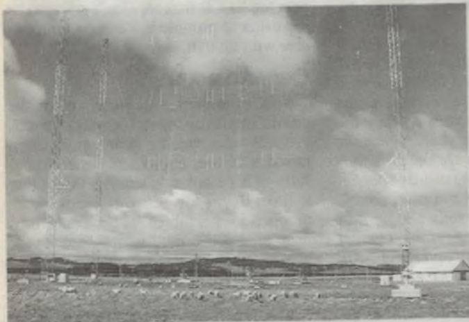
The transmitter building and towers of Radio New Zealand International at Rangitaiki. The building houses a 100kW transmitter.
