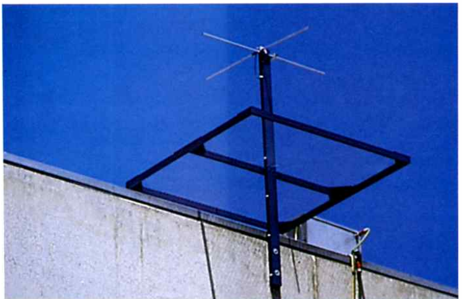
Photo 4: A turnstile/reflector or TR antenna for weather satellite reception, installed on a science building at Hobart college.
