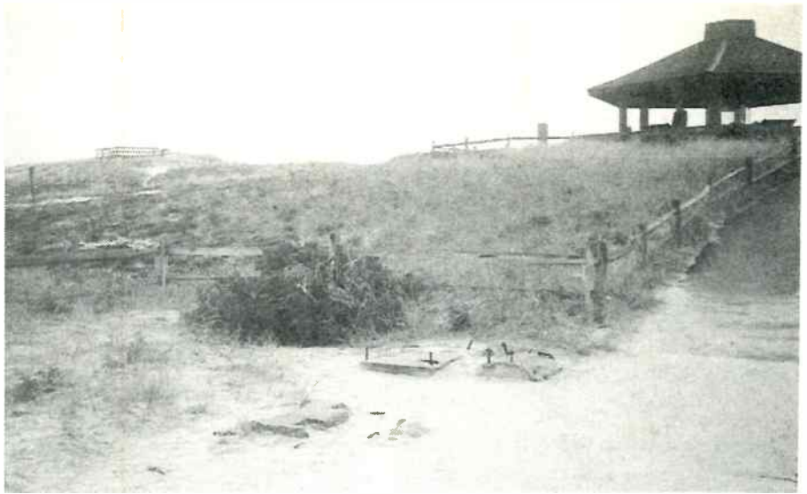
Fig.3: The site of the second Marconi transmitter near Harbour Grace, which replaced the first one — destroyed by a cyclone shortly after its erection. The building on the right houses a model of the installation. Adjacent to it is a memorial obelisk and, to the far left, a viewing platform. (Photo by 'Blue' Easterling).
