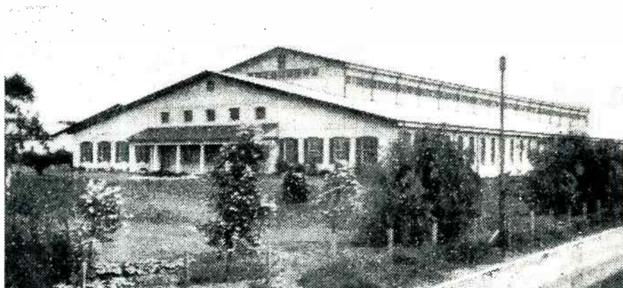
One of the two main buildings on the Ashfield site when AWA purchased it in the middle of 1930. It became known as the 'Radiola' building, and produced huge numbers of radio and television receivers. (From Wireless Weekly, April 10, 1930).
