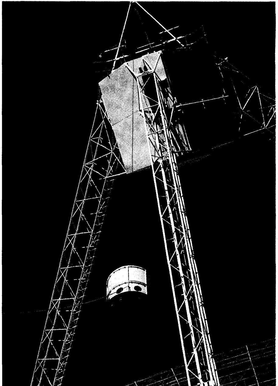
The new Multibeam Receiver module is winched up to the enlarged focus cabin of the Parkes radiotelescope. The array of 13 feed horns is visible at the bottom. (Picture courtesy Elly Hakvoort, ATNF)
