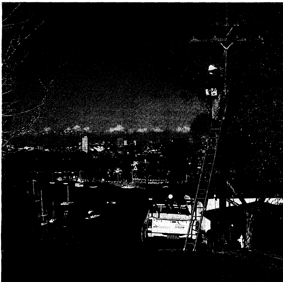
Installing aerial broadband cable in Longueville, a harbour suburb of Sydney. Optus Vision is using SA transmission products including amplifiers, line extenders and multimedia taps. Visible in the background is Sydney harbour and the city skyline. (Courtesy Scientific Atlanta)
