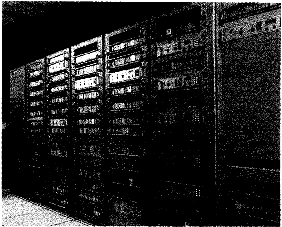
A typical broadband system headend, in this case manufactured by Scientific-Atlanta. The racks of electronics manage the distribution of signals to the HFC network. (Courtesy Scientific-Atlanta)
