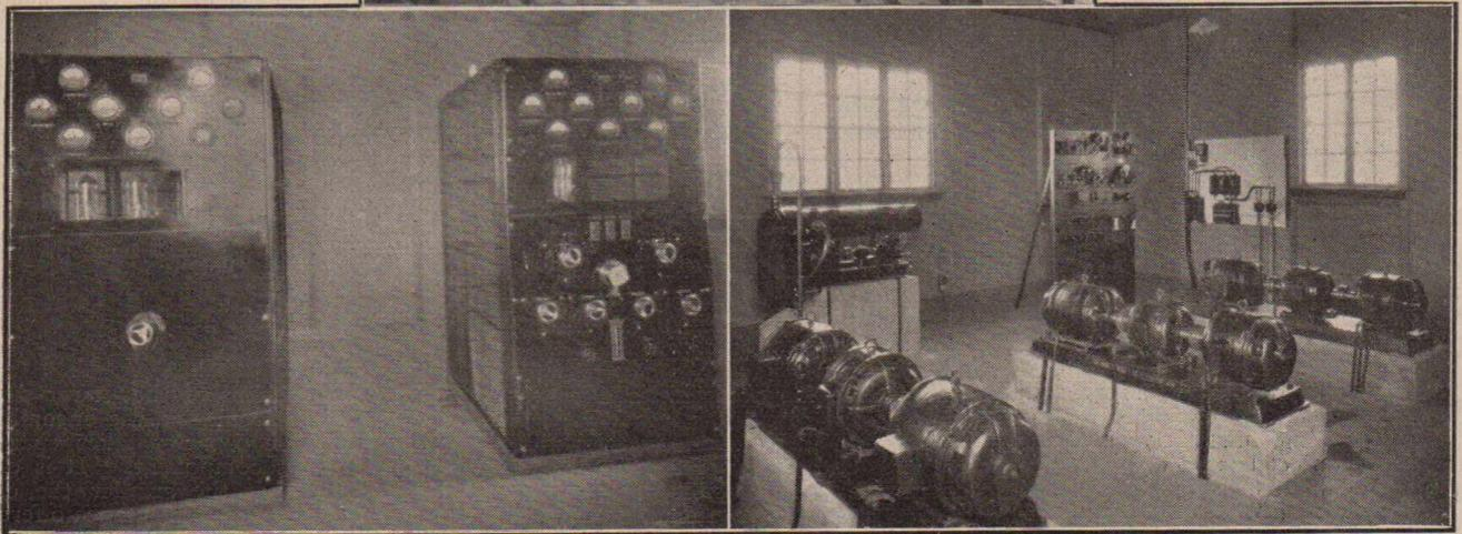
A view of portion of the 4BH studio (top). At the left is shown the modulator and the oscillator-amplifier stages of the transmitter. The right hand picture shows the power supply equipment, with the water-cooling pump system in the left background.
