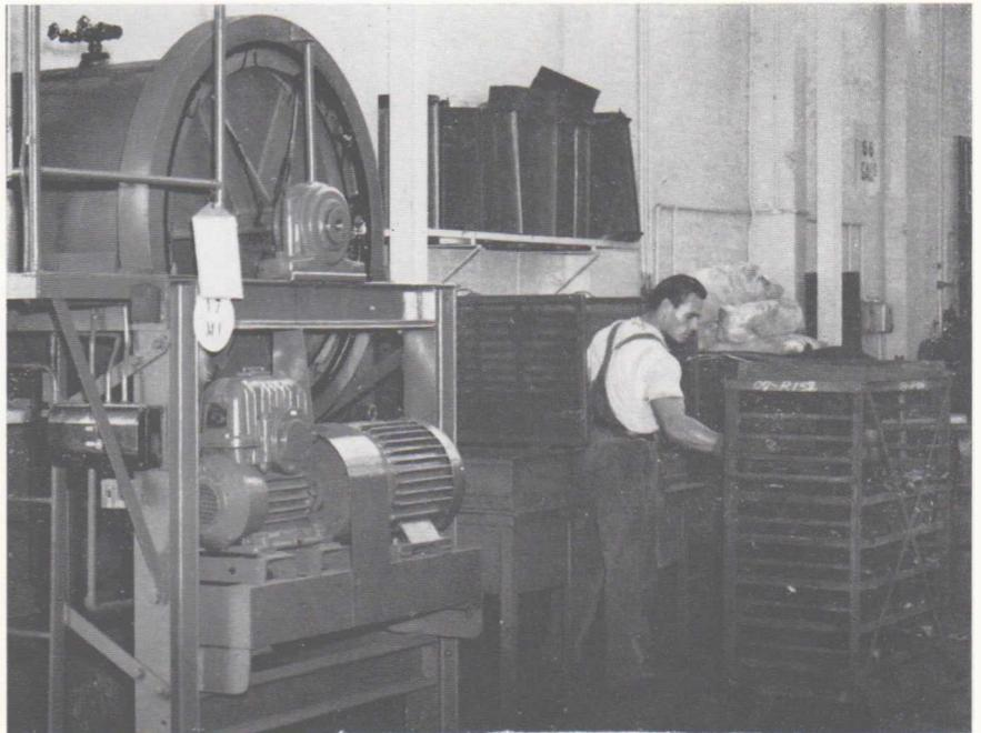
"Ball Mill" and filters used in preparation of ferrite powders.
