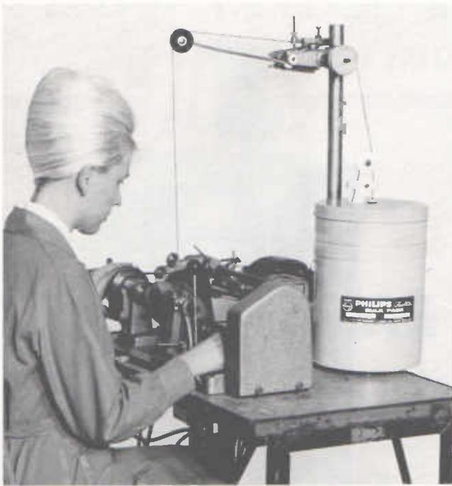
Fig. 2. Philips Bulk Pack used with dynamic wire tensioner which has had the spool replaced by a small Vee pulley.
