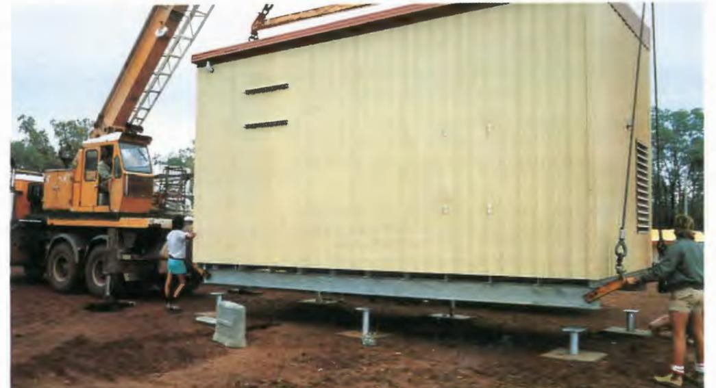
Transmitter building being placed in position - 4CH.
