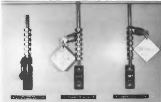
*Matrix arm isolation switch fitted with cradle and padlock..*
