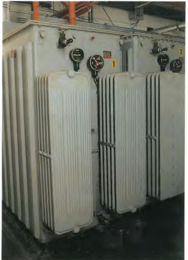
*Typical oil filled transformers 250kW transmitter*
